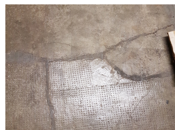
F.4 Joint de fissures
