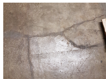
F.4 Joint de fissures
